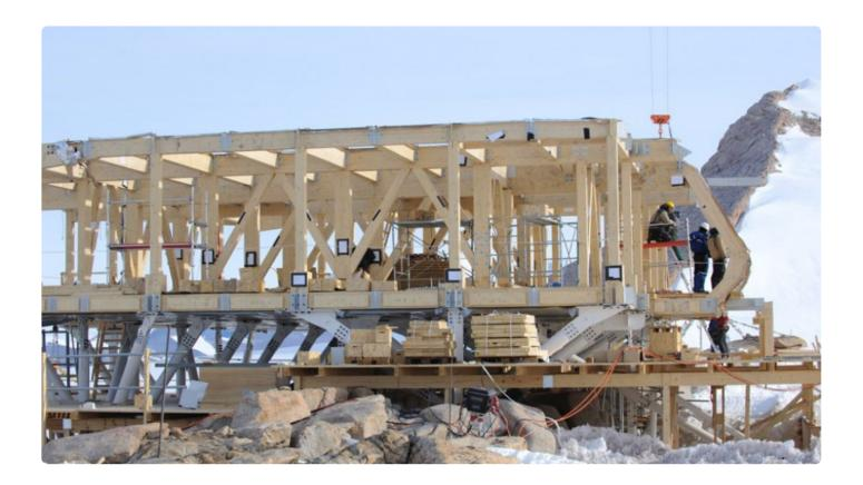
The C-shaped wooden side beams have now all been mounted. Next step involves tackling the exterior metal panels, as soon as the weather permits to do so.
