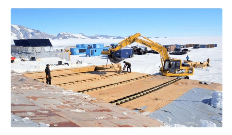
Already several weeks into the new season, the old garage on the north side of the station is in the process of being torn down while the anchor points for its replacement are being installed.
